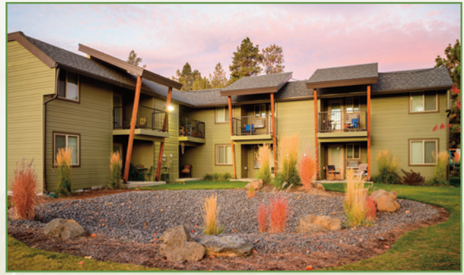
Crest Butte Apartments, Bend Oregon -- Viridian Management (Manager) /Chrisman Development (Developer)
